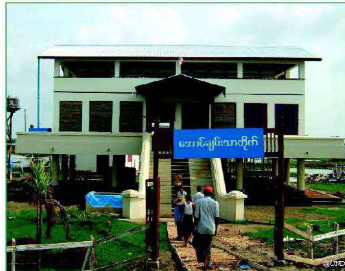
A monastery elevated on posts, piles above flood level so that the community can use it as a shelter during a flood.
